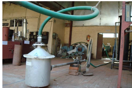
Fig 3.3: Fabric filter incorporated to further clean the producer gas
